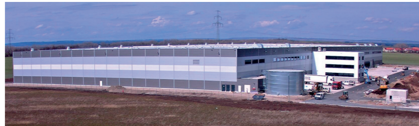
The new logistics center of Berger Logistik GmbH in Erfurt-Stotternheim. Photo: Berger Logistik GmbH , 04/2018
